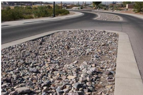
**A median in this road in Las Cruces allows runoff from the asphalt to flow into the median and soak into the ground below the rock.**
