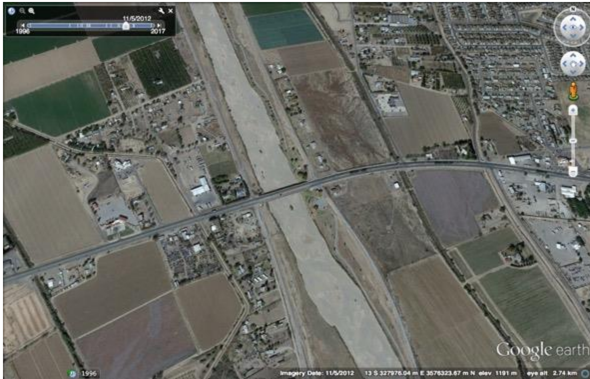
FIGURE 6. Water depth at Elephant Butte Irrigation District Picacho Bridge gauge during 2012 (upper panel) and Google Earth imagery of Rio Grande at Picacho Bridge on 5 November 2012 showing a dry river bed (lower panel). The Picacho Bridge is about 2.3 km upstream of the LCWTF discharge.
