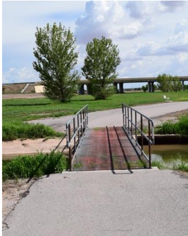
FIGURE 5. Las Cruces wastewater drain and Rio Grande floodplain.
