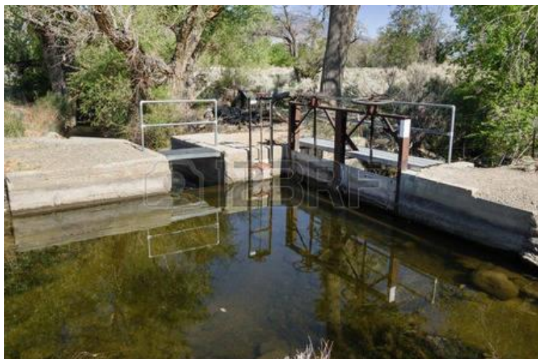
FIGURE 10. Control structure splitting flow between channels. (Source: http://us.123rf.com/450wm/pancaketom/pancaketom1406/pancaketom140600016/29073241-water-diversion-structures-to-control-the-flow-of-water-from-an-irrigation-canal-in-the-owens-valley.jpg?ver=6 )
